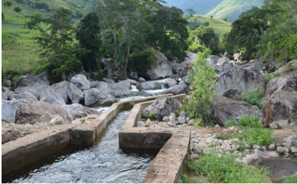
Figure 1-8. A photo showing diverted water from Lichenya River directed to the siltation chamber of Bondo 1. (Source: Photo by the Author)
