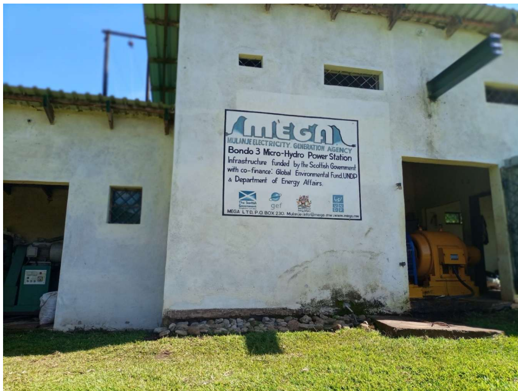
Figure 1-14. A photo showing the power house for Bondo 3 which also serves as the control room for all the power plants. (Source: Photo by the author)
