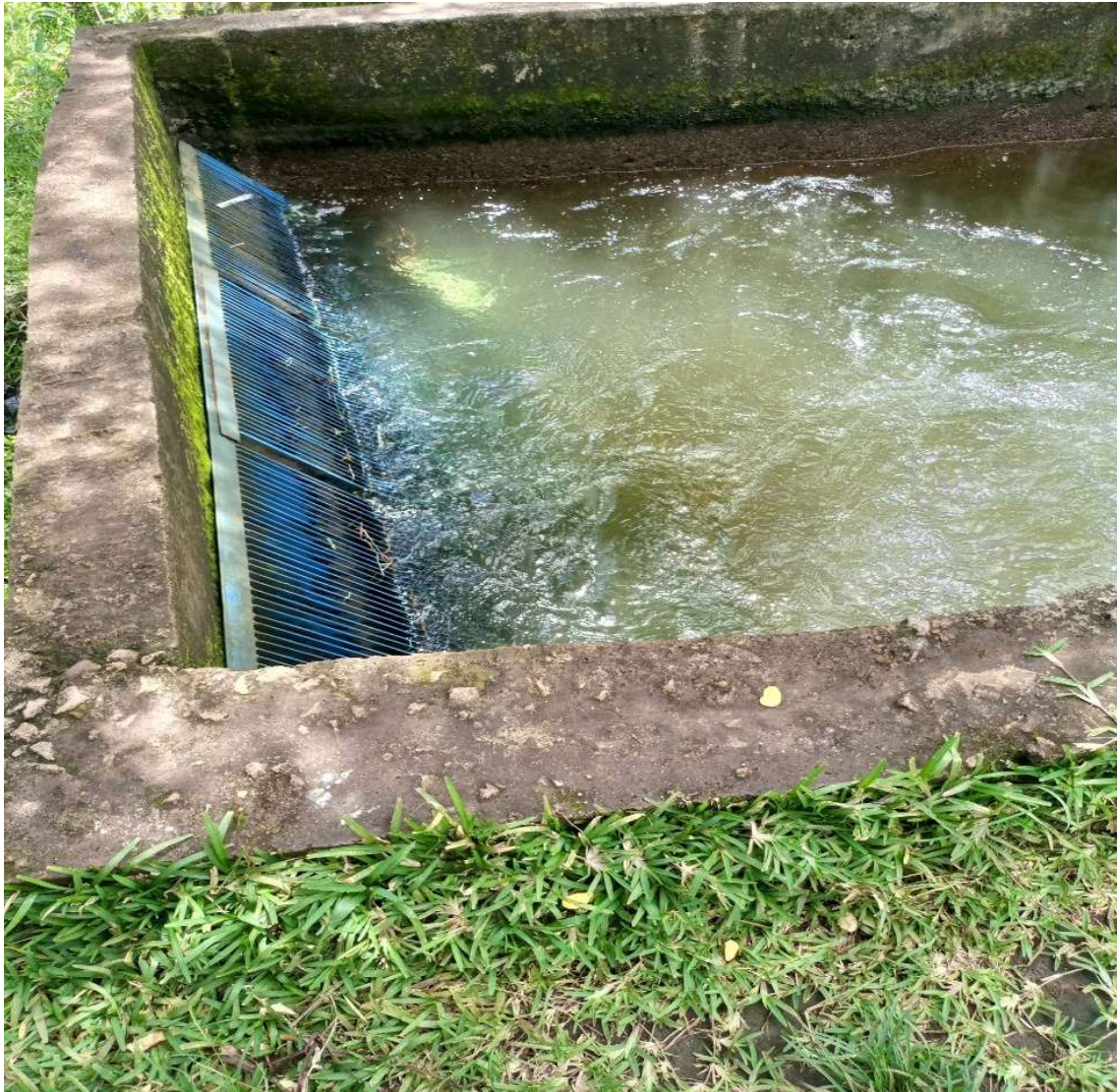
Figure 1-10. A photo showing the forebay on Bondo 1. (Source: Photo by the Author)
