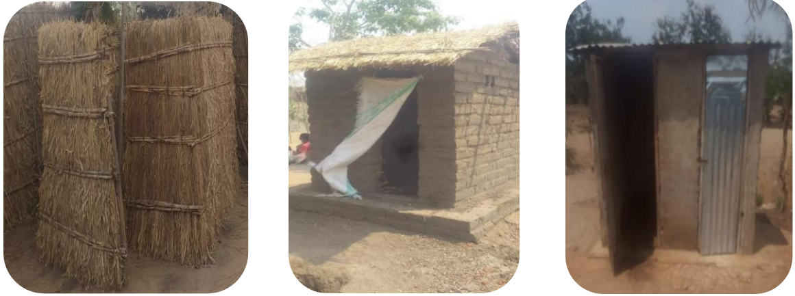
Figure 15 Type of Simple Pit Latrines available in Balaka four years after ODF certification
