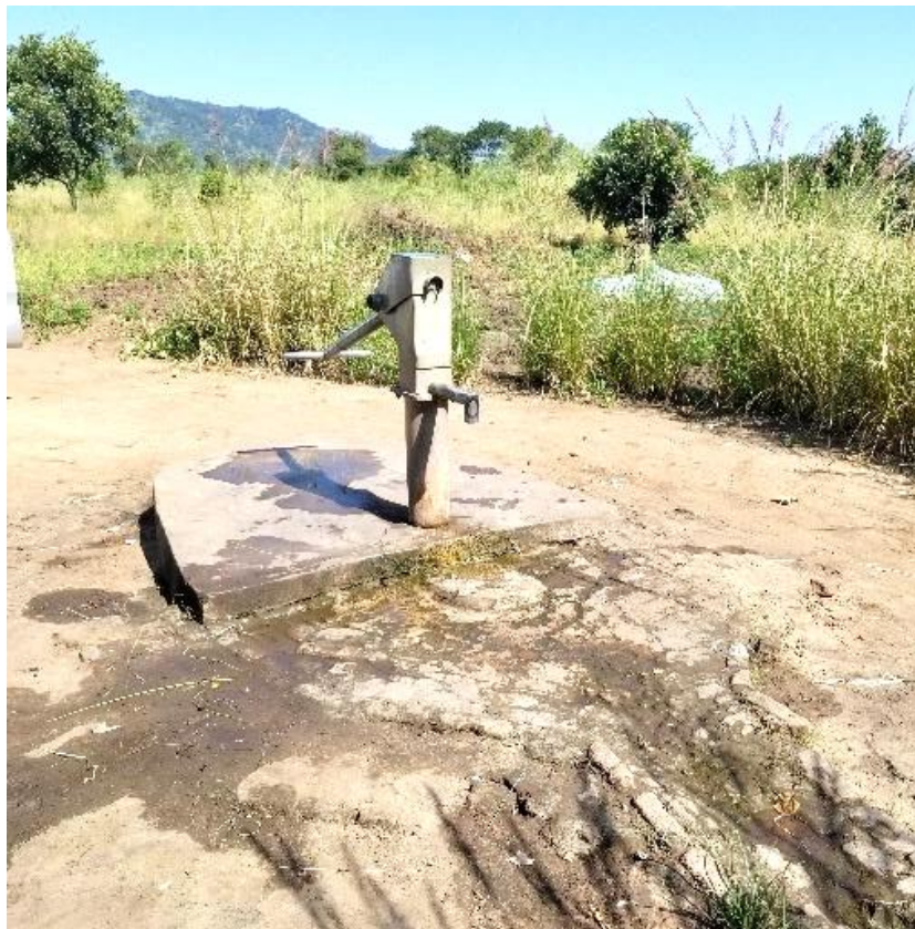
Figure 4-8: Apron made of bricks and plaster
