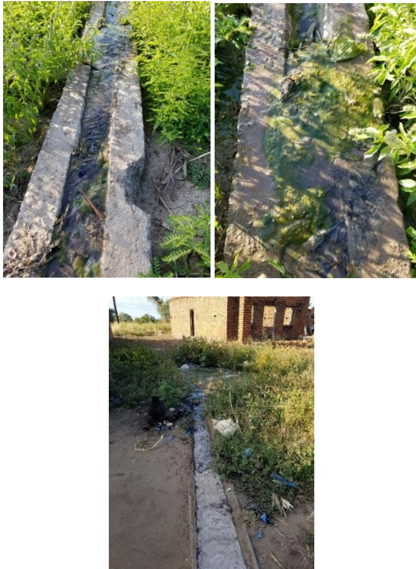
Figure 4-6: Poor waterpoint surrounding
