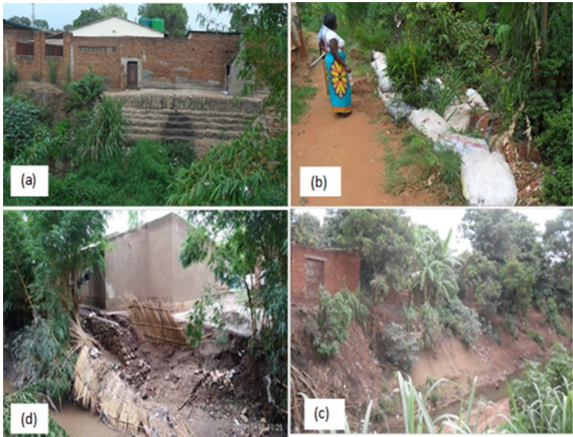
Figure 27: Some of the building protection measures
