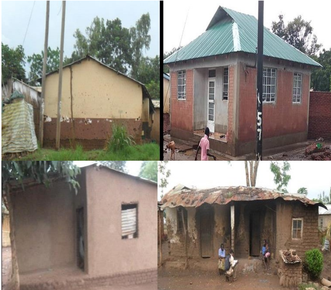
Figure 16: Some of the buildings in the study area
