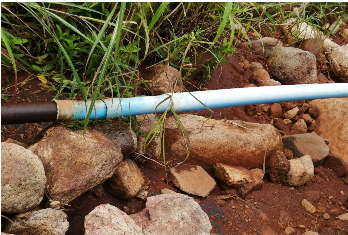
Figure 13: Maintenance using old materials.
