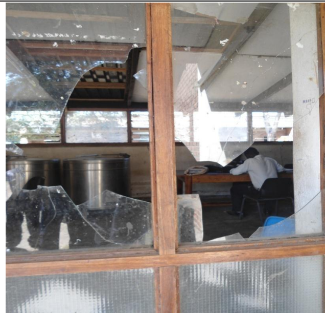
Figure11: Student N: ' students angered with new rules of the new regime '...photo showing broken glasses on the Library entrance door
