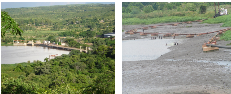
Figure 2. The water intake dam at Nkula Falls on the Shire River (left); heavy siltation (right).
